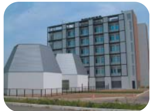
▲ Next-Generation Post-Genome Research Building
