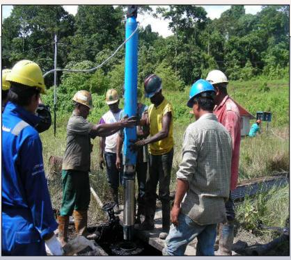
THE USE OF ESP (ELECTRIC SUBMERSIBLE PUMP/175 TO REACTIVATE SUSPENDED WELL
