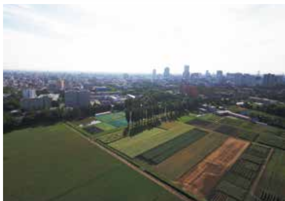
An aerial drone image of the Sapporo Campus
