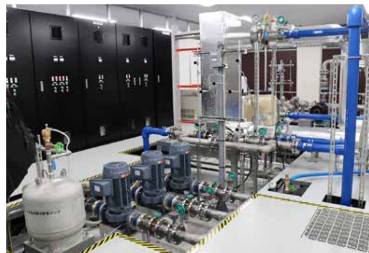
The water-cooling system.
